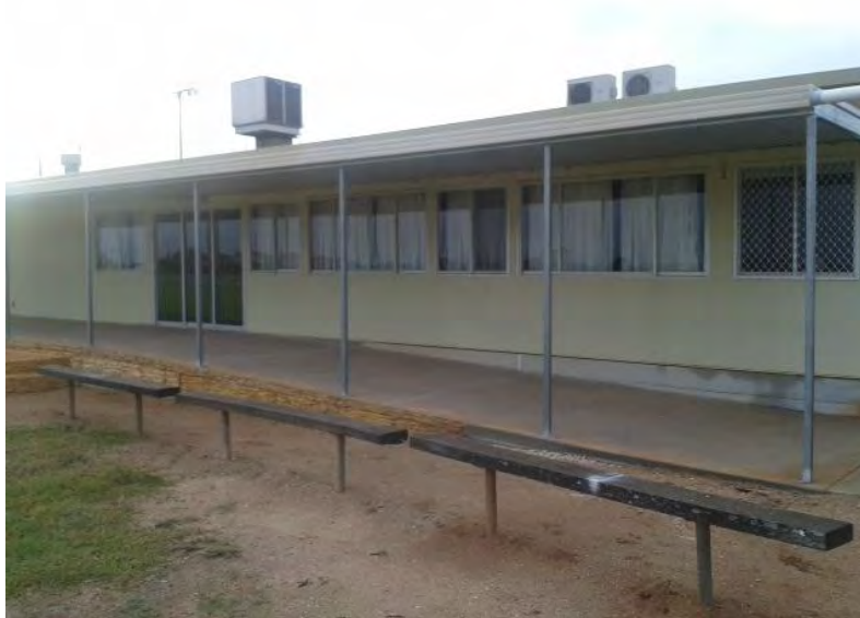
The completed access ramp at the Western United Tigers Football Clubrooms, Penong.
