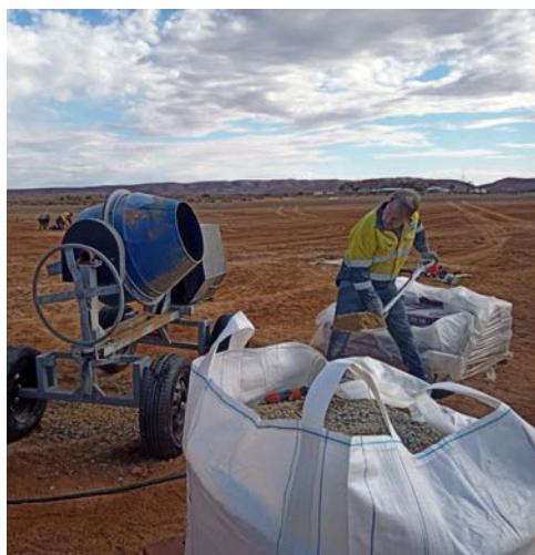
A-PAPI installation work starting at the Airport
