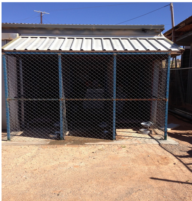
The new dog detention facility at Andamooka.
